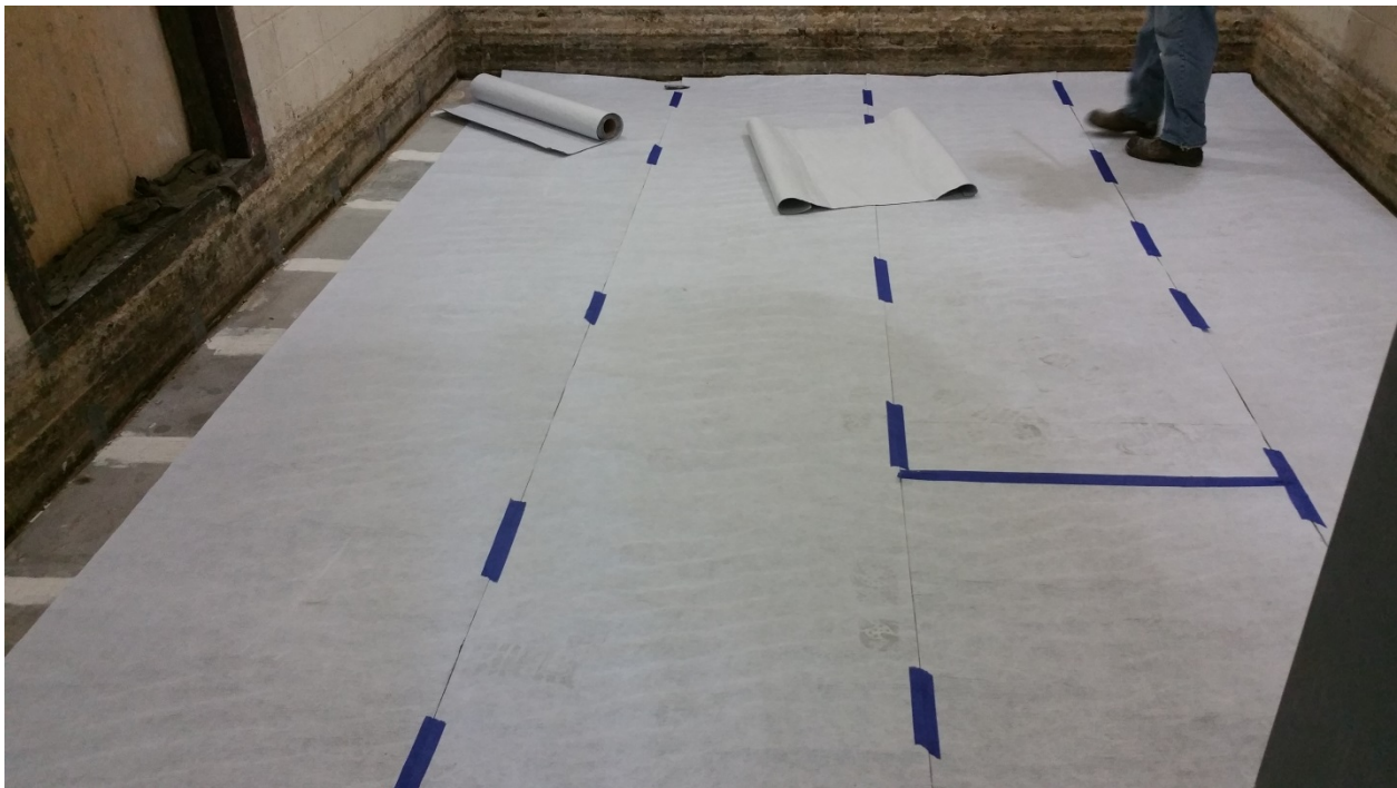
Figure 2 – Fracture Ban™ 90 membrane placed over concrete slabs.
